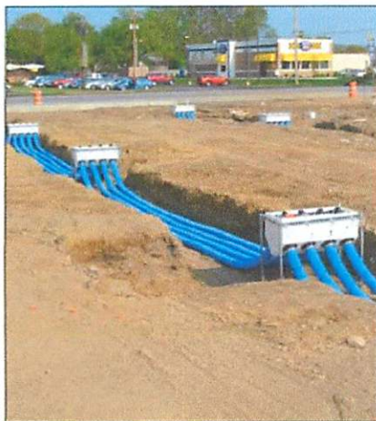
Figure 6. Multilayer underground fuel pipe with Kynar Flex® PVDF as inner contact layer. Photo courtesy of OPW Fuel Systems.
