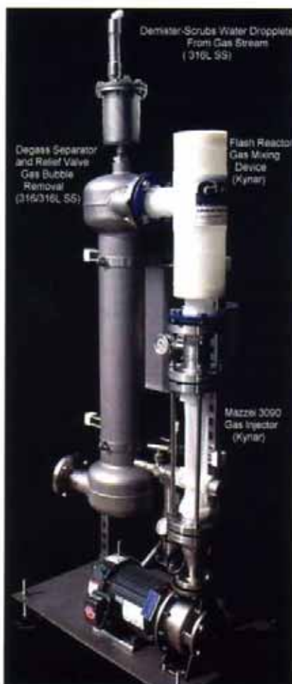
Mazzei ozone PVDF Injector, stainless steel demister and stainless steel separator in cooling tower ozone system that has helped to reduce water treatment costs $70,000 per year.
